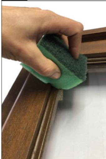
Even though glazing beads are pre-painted in the factory, with prolonged exposure to the elements they are often the first part of a window or door to show signs of deterioration.
